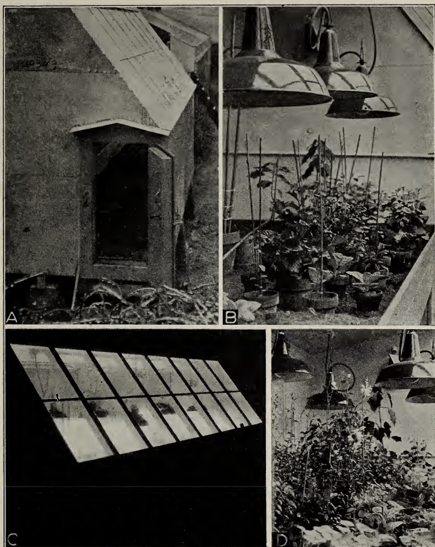
FIGURE 124. A, End view photograph of the new type greenhouse showing the refrigerator type of door and the method of supporting the house on cement pillars. C, Night view through the storm sash. B, Plants inside the house on December 29. D, Same plants taken February 9, or 42 days later.
